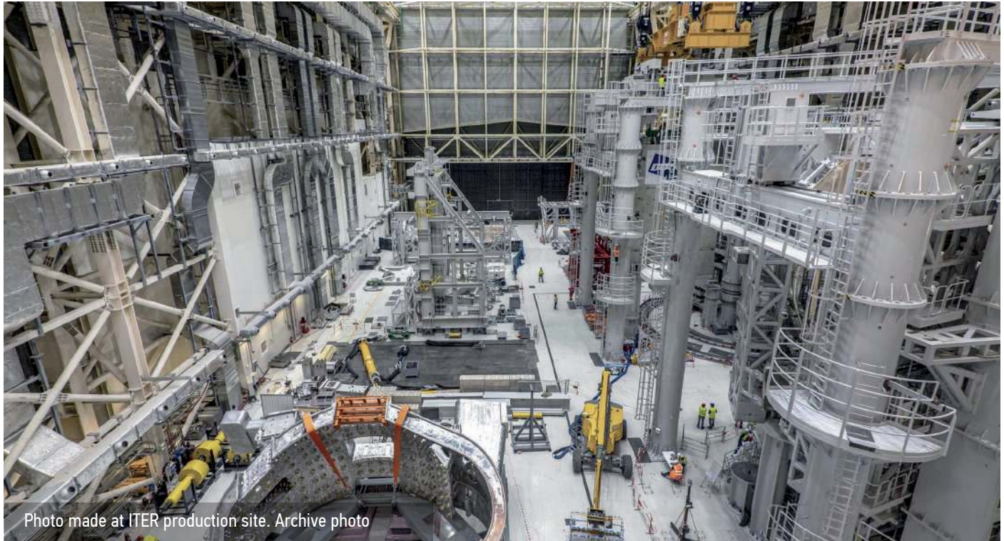
Photo made at ITER production site. Archive photo
